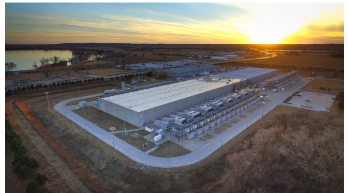
Google Data Center
